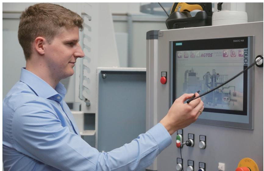
Christopher Fritz Dietrich, Project Engineer for factory planning and organisation, demonstrates the ease of operation on the clearly arranged panel
